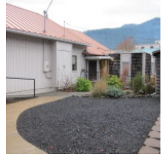
Back sidewalk and landscaping
